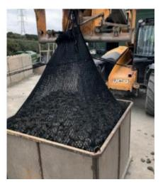
4. Two workers will be needed for this, and the following work step. Pull the tying rope around the AquaRockBag in opposing directions as shown below.
