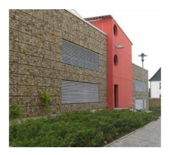
Made of electro-spot-welded, steel-wire mesh grids with the facing panel and side panels as one continuous piece bent on each end. The clean lines and small rectangular openings provide a premium aesthetic while allowing flexibility in fill material. The baskets are shipped in their 3D form and filled on the ground and then placed on the included wall brackets utilizing the mounting hooks on the back of the baskets.
